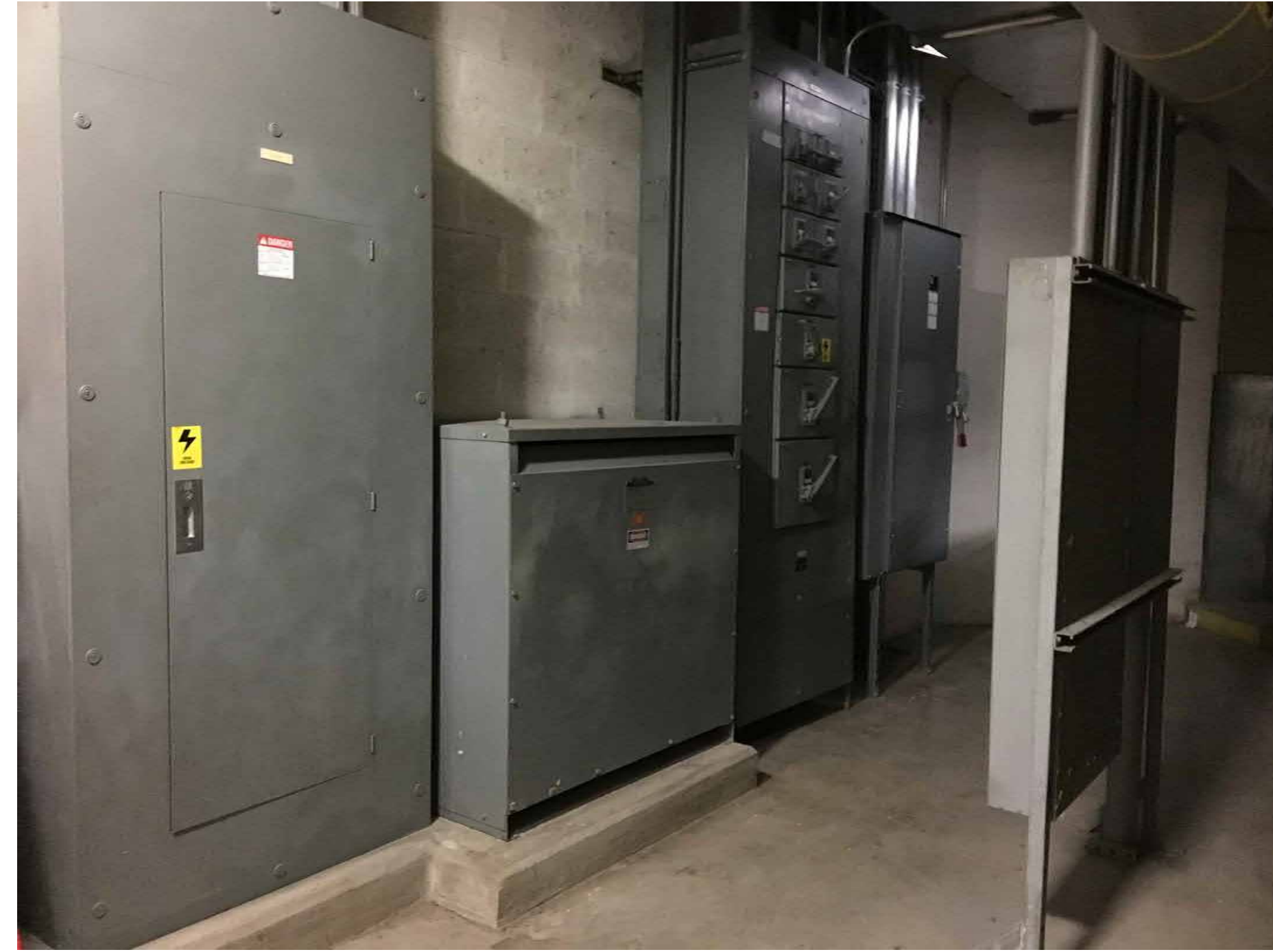
2 EXISTING - 6TH FLOOR ELECTRICAL DISTRIBUTION LINEUP NTS
