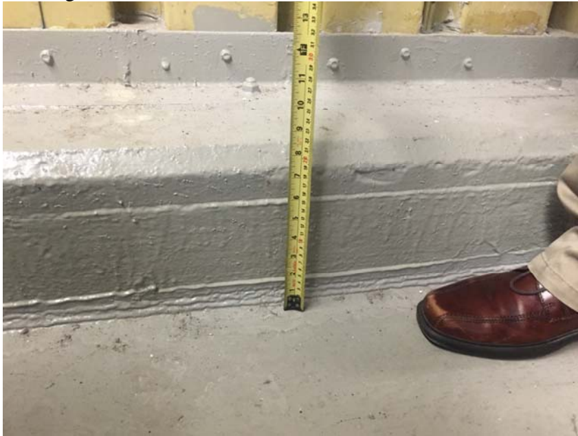
Existing AHU curb:
