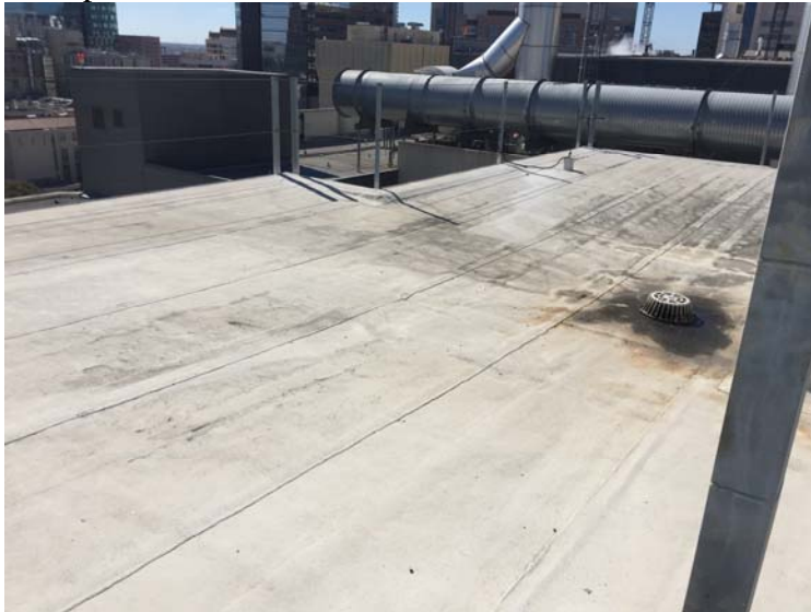
Roof penetration area:
